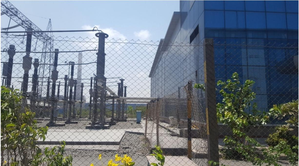
220 KV and 400 KV GIS substation is available in Essar, Hazira. Total 6 bay is there. 2 bay for Gen, 2 line bay , 1 bus coupler bay and 1 CT, PT bay.
